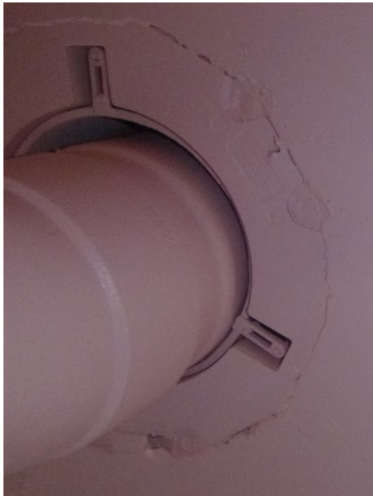
Figure 25c: Thin painted on collar shell and intumescent, refer to Table 17c
