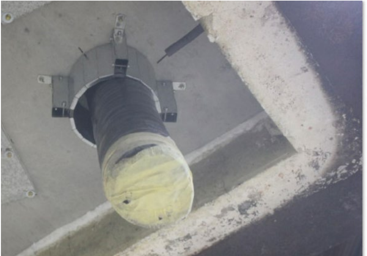
PHOTOGRAPH 2 – EXPOSED FACE OF SPECIMEN 3 PRIOR TO TESTING
