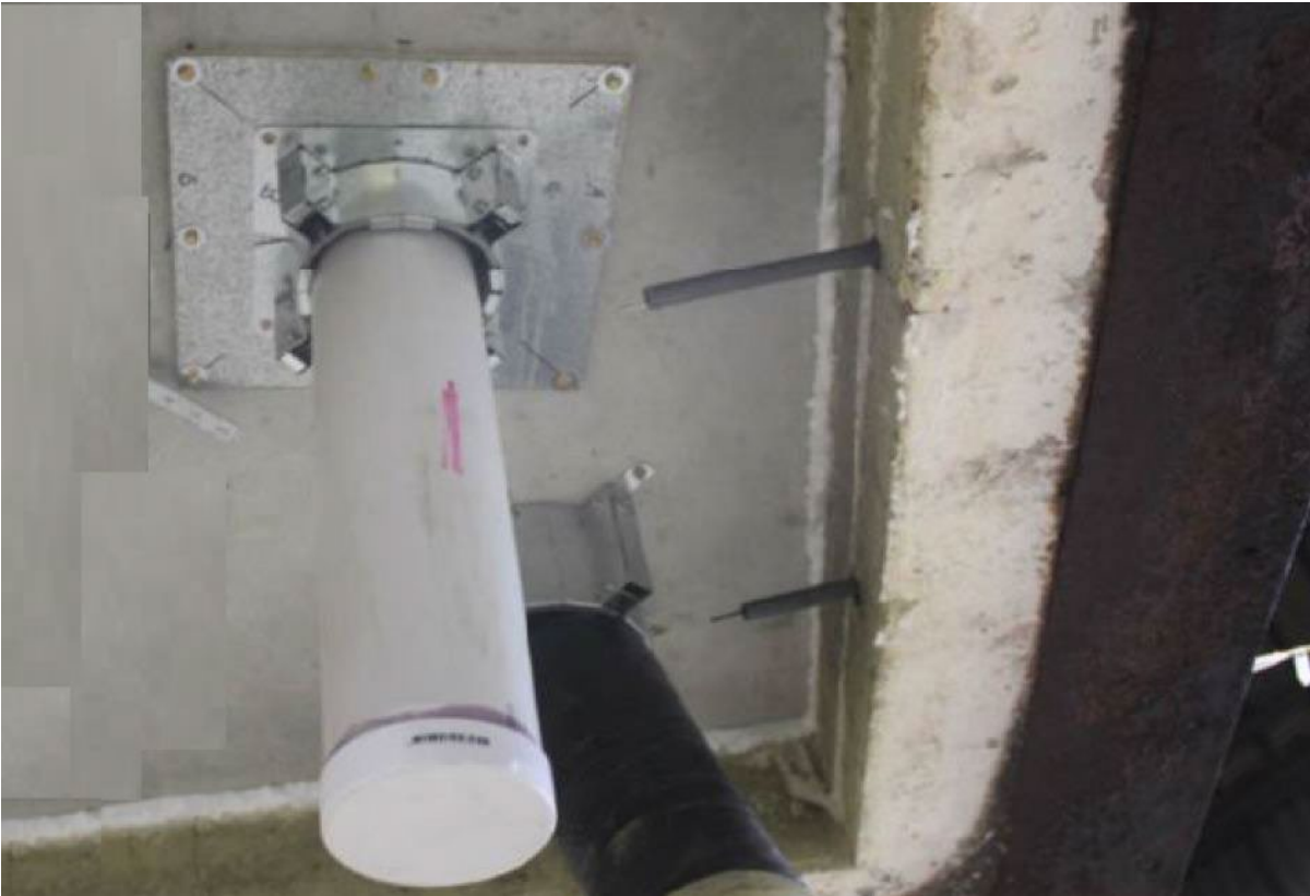
PHOTOGRAPH 1 – EXPOSED FACE OF SPECIMEN 1 PRIOR TO TESTING
