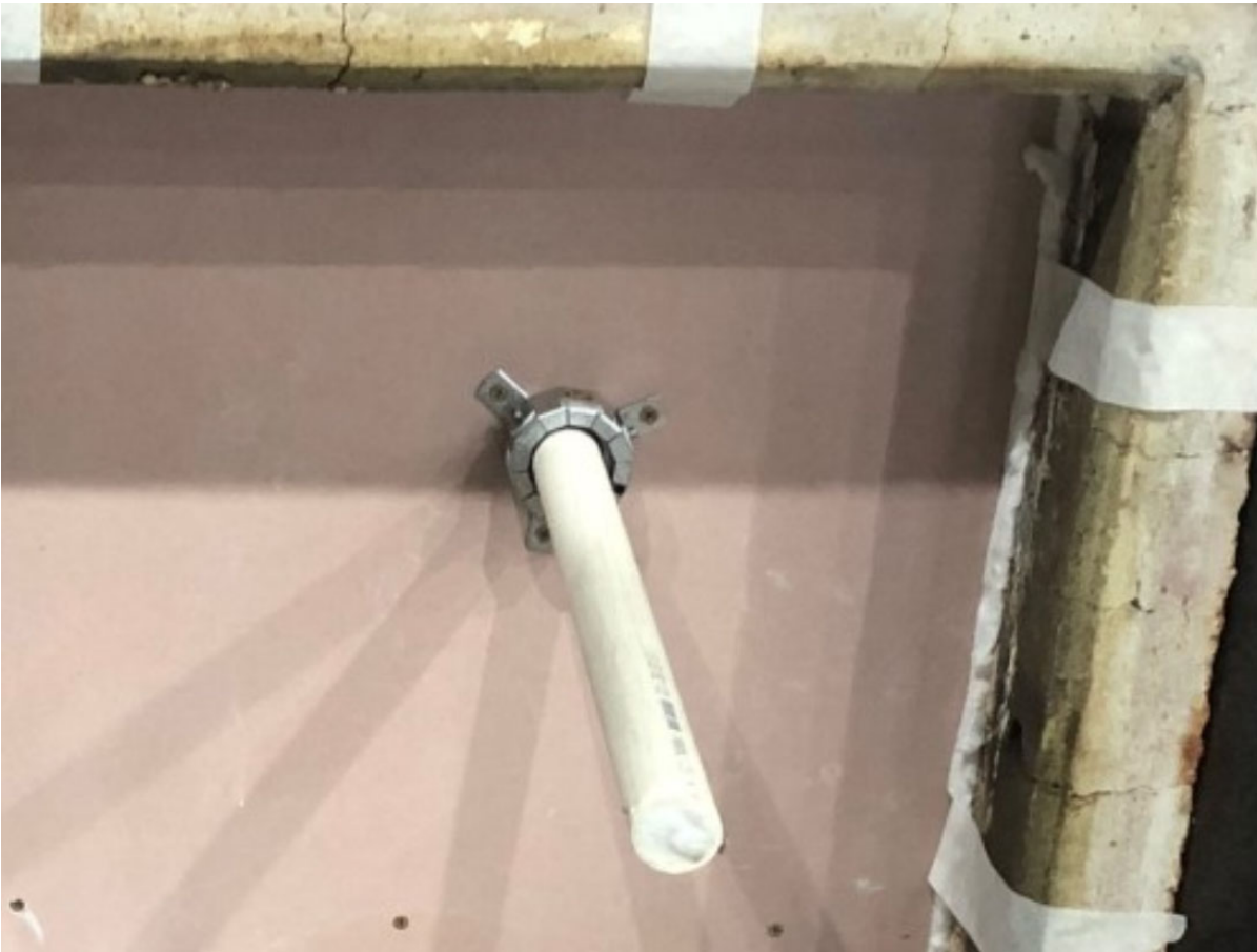
PHOTOGRAPH 1 – EXPOSED FACE OF SPECIMEN 1 PRIOR TO TESTING
