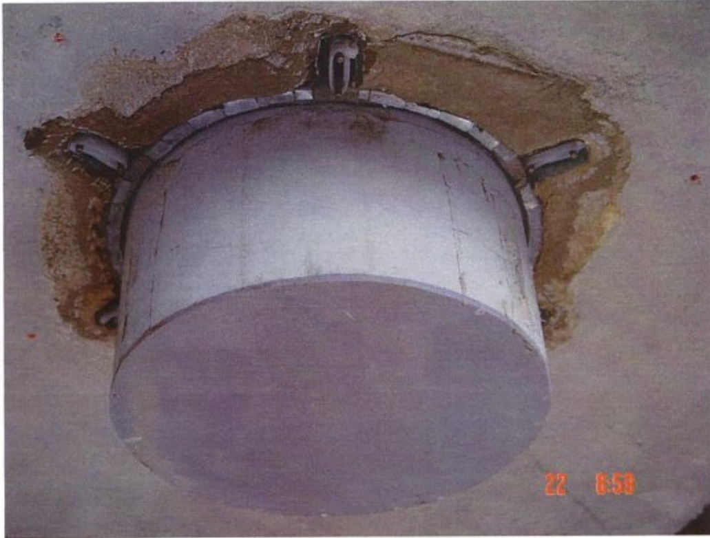
Photograph 1 - Specimen (exposed side) prior to testing.
