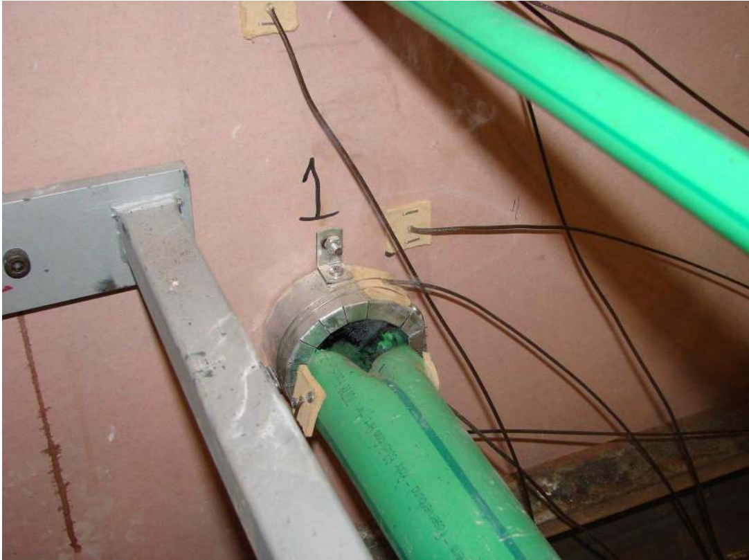
Photograph 5 – Pipe #1 after 170 minutes of testing
