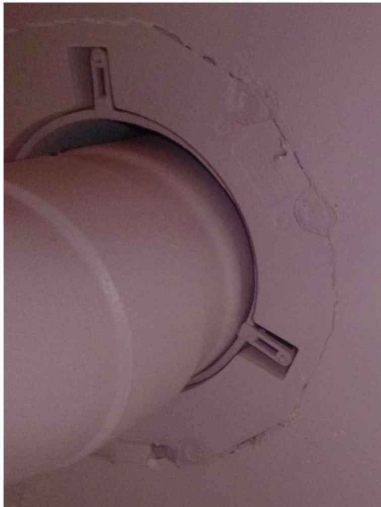
Figure 25c: Thin paint on collar shell and intumescent, refer to Table 17c
