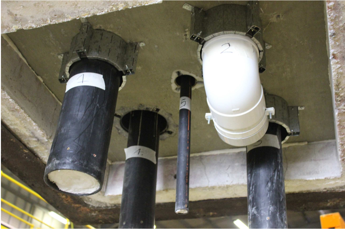
PHOTOGRAPH 1 – EXPOSED FACE OF SPECIMENS PRIOT TO TESTING
