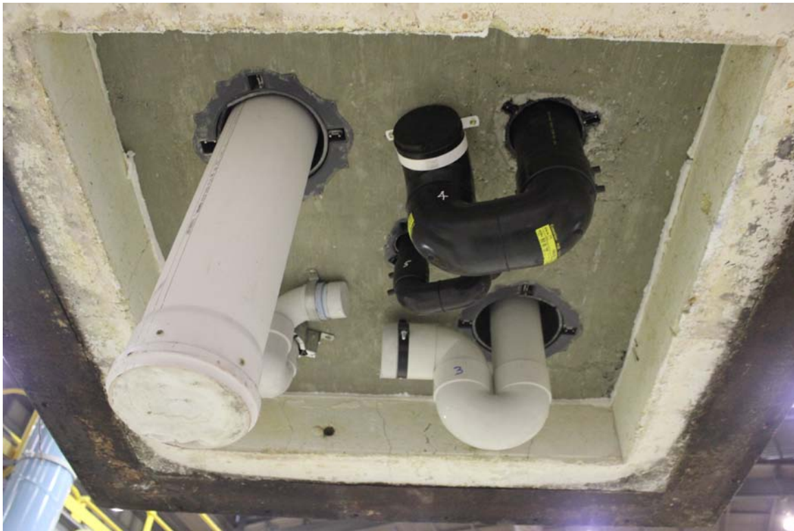
Photograph 1 – Exposed face of the specimen prior to testing
