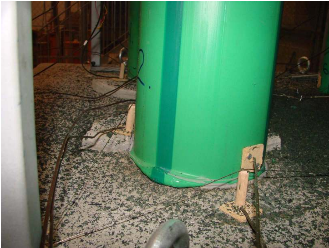
Photograph 7 – Pipe 2 after 200 minutes of testing
