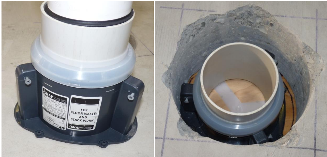
Unexposed Face after Grouting and 35 mm thick Screed Topping
