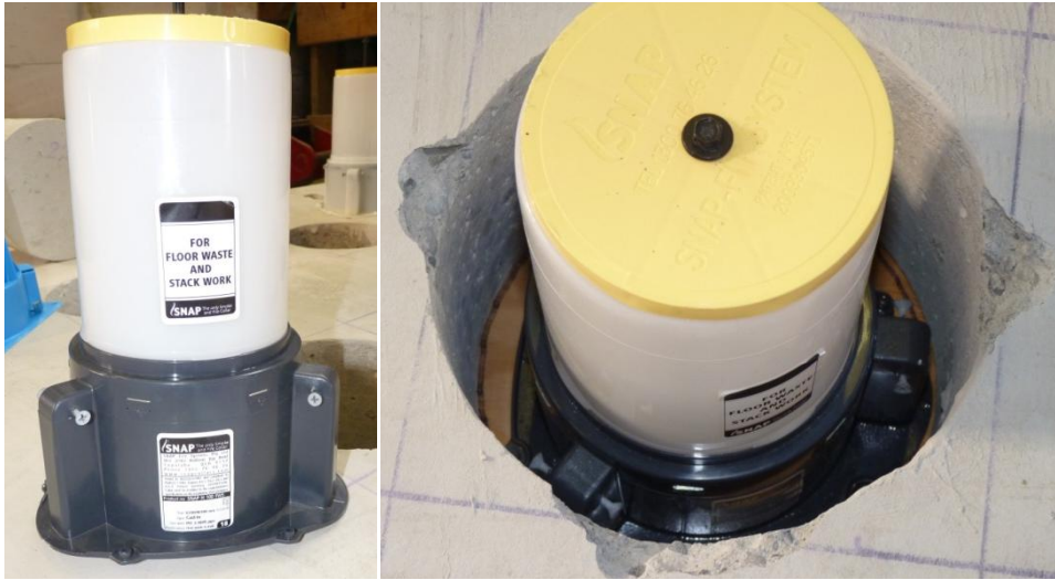
Unexposed Face after Grouting
